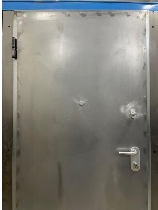
Figure 1: Door in the as delivered state before the start of the test, sectioning the two rooms.
