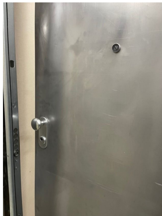
Figure 2: Door in the as delivered state before the start of the test, sectioning the two rooms.
